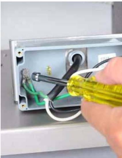
**Step 12:** Using the splice provided, crimp together the power cord's white wire with the motor cord's white wire.
