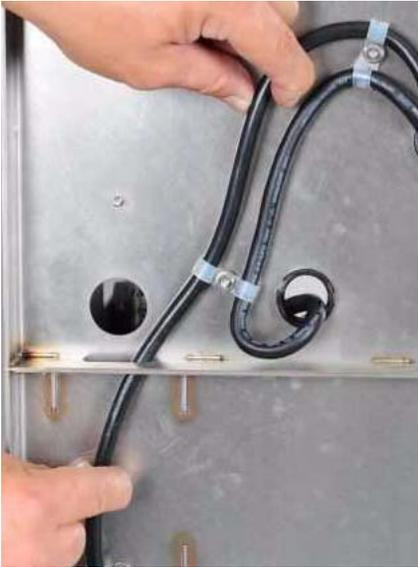
**Step 10:** Reinstall the nuts, washers and cable clamps under the frame.
